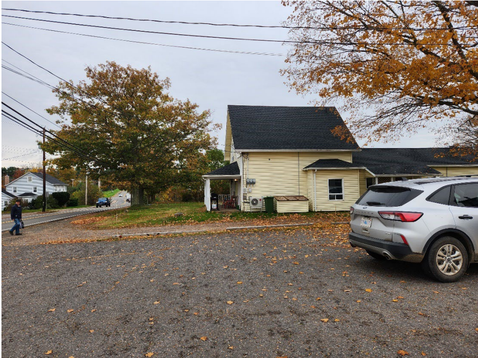
Neighbouring dwelling to the west
