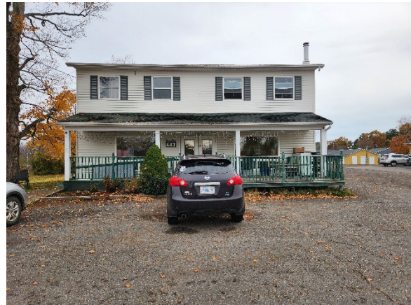
Figure 2: Existing Building and Parking
