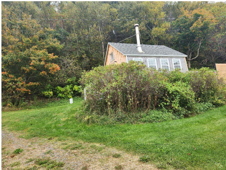
The cabin encroaching onto the adjacent property
